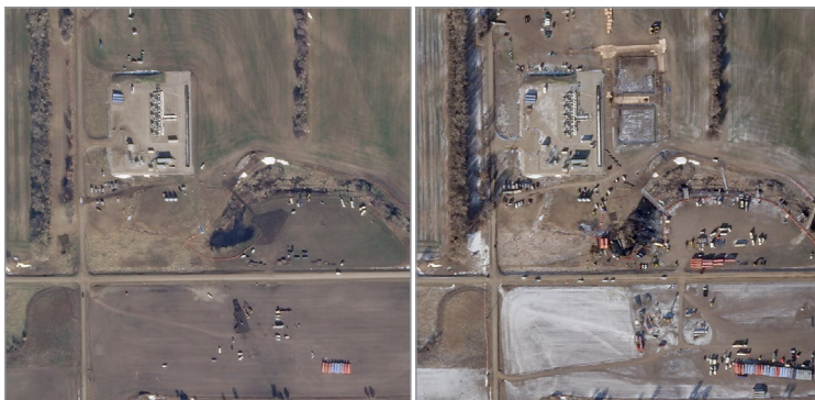
Keystone pipeline spill in Edinburg, North Dakota • Nov 2, 2019 and Nov 7, 2019
